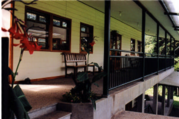
MVI Library with a classroom and the lab below.
